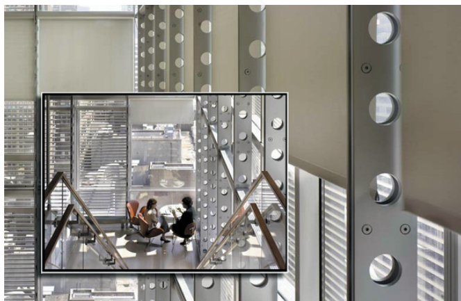
To control daylighting for maximum comfort and energy efficiency, computer-controlled shades respond to changing exterior conditions. (Photo Renzo Piano Design Workshop)
